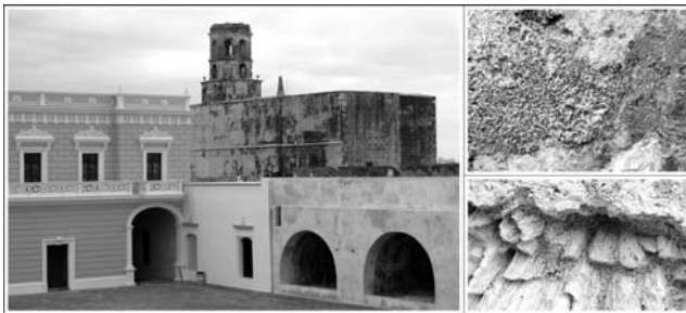
Figure 10: San Juan de Ulúa recent restoration and the masonry – with hard coral substances in the walls (photos Guillén, 2013).
