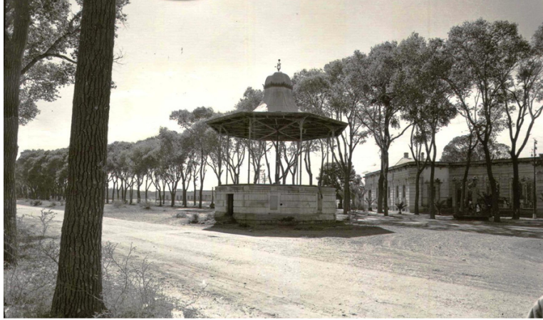
Figura 6. Calzada Arellano, ca. 1903
